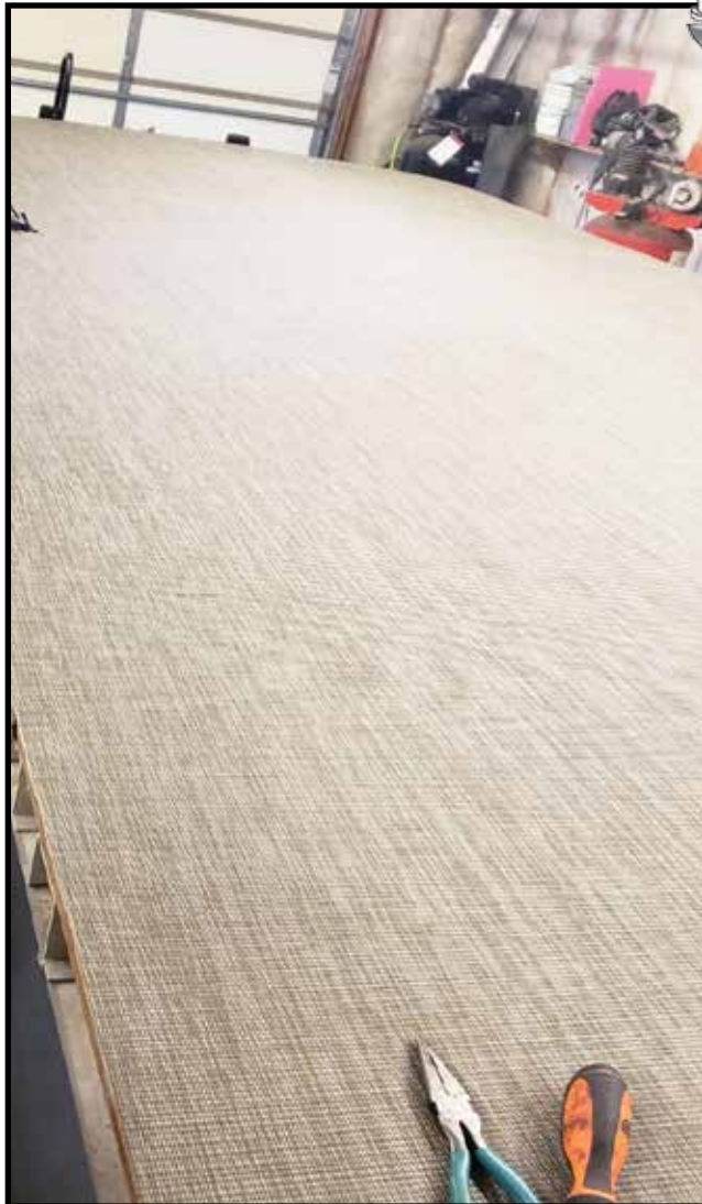
New woven flooring being applied
